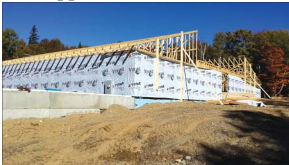
UNDER CONSTRUCTION – House in the Woods, a retreat for veterans and their families, is taking shape in Lee. The program has served over 500 veterans since 2010. (Deanna House photo)
